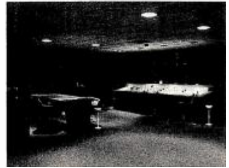
This is one of four production control rooms in the Metromedia center. Each commands three video-tape recorders and two telecine islands. Announcer booths and client viewing rooms are attached to each control room.
